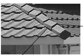
Two "C" channels stacked on top of the Divine panel batten channels.
