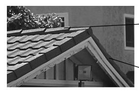
Two "C" channels stacked to form a 5" wide ridge beam.
